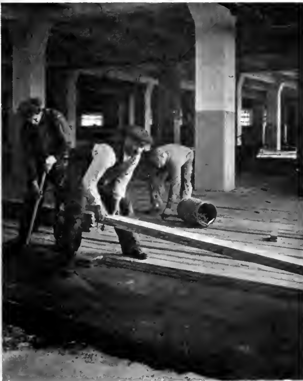
METHOD OF LAYING THE WOOD FLOORING
